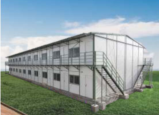
Shapoorji Pallonji & Company Pvt Ltd G+1 Accommodation Structure Back-to-Back Arrangement
